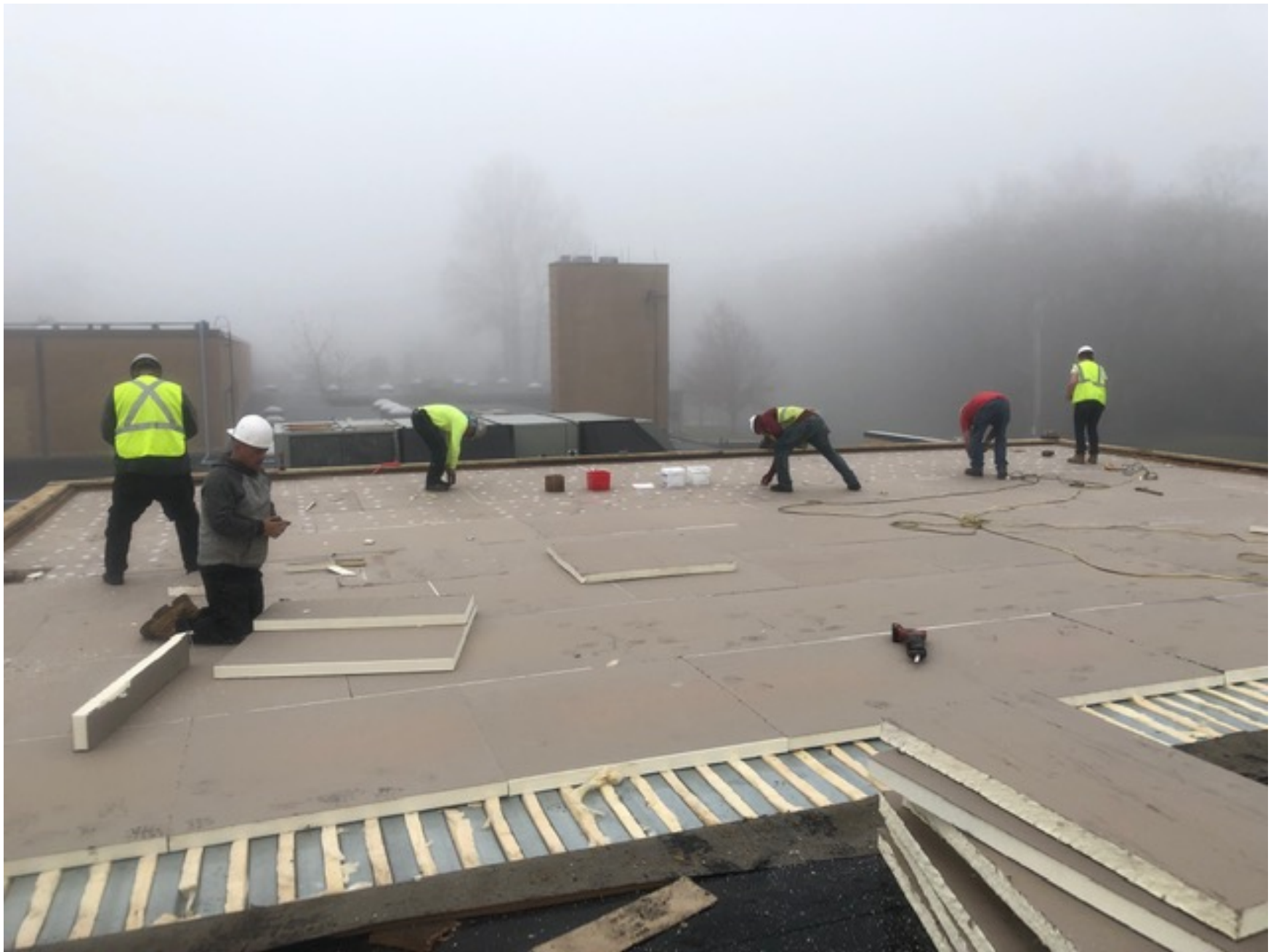
MS/HS Roofing replacement
